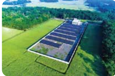
Solar Mini-Grid Project at Jamalpur
