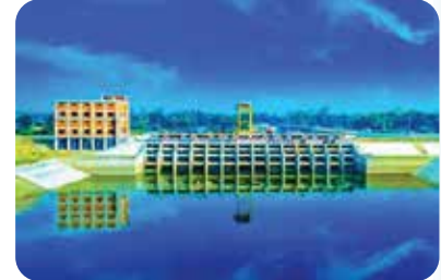
Talimnagar Pump House, Pabna
