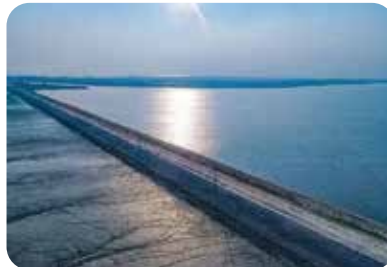
Musapur Clouser construction at Noakhali
