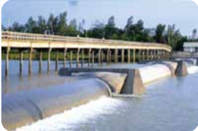
Rubber Dam construction Project at Cox's Bazar
