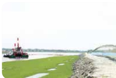
Dredging project to improve navigability at Mongla - Ghasiakhali, Rampal
