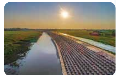
River Bank Protection at Charfassion, Bhola
