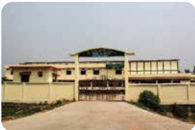
Cold Storage construction at Kurigram
